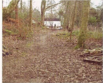
Access road for the National Lake District Parks Authority. Site before construction pictured above.
