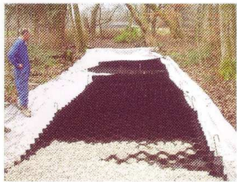
Cellweb during installation.
